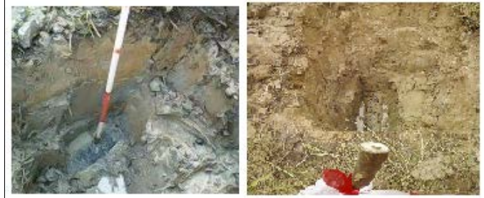
Fig. 2: An excavated point revealing utility (pipeline) nature on identification.
